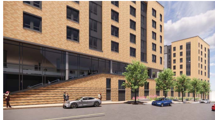
STREETVIEW FROM E. WOOD ST.
