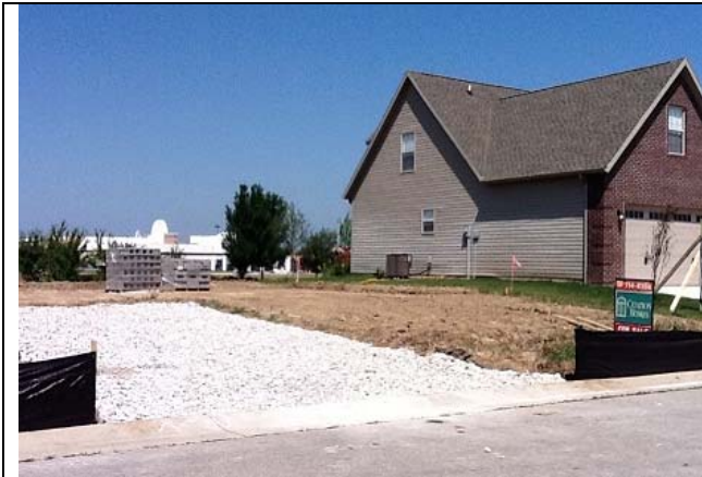
Construction drive and silt fence properly installed.
