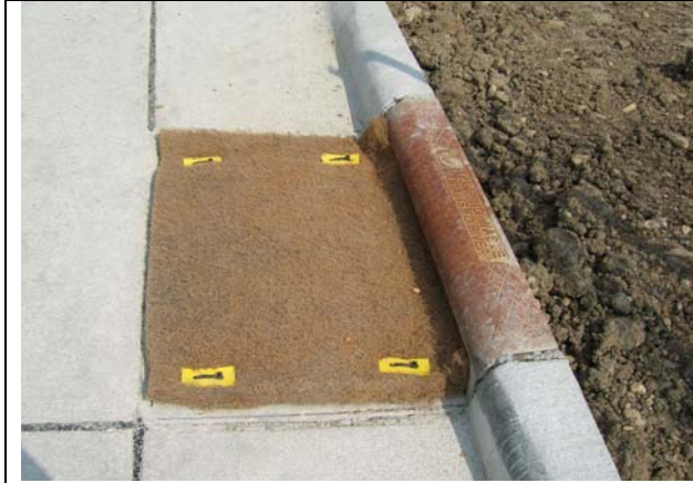
Straw inlet mat properly installed over a storm inlet.
