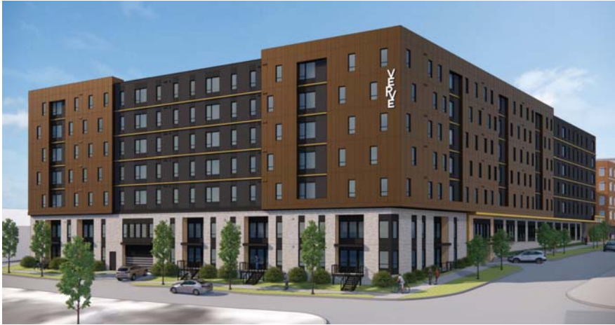
VIEW FROM THE NE ON WOOD STREET
