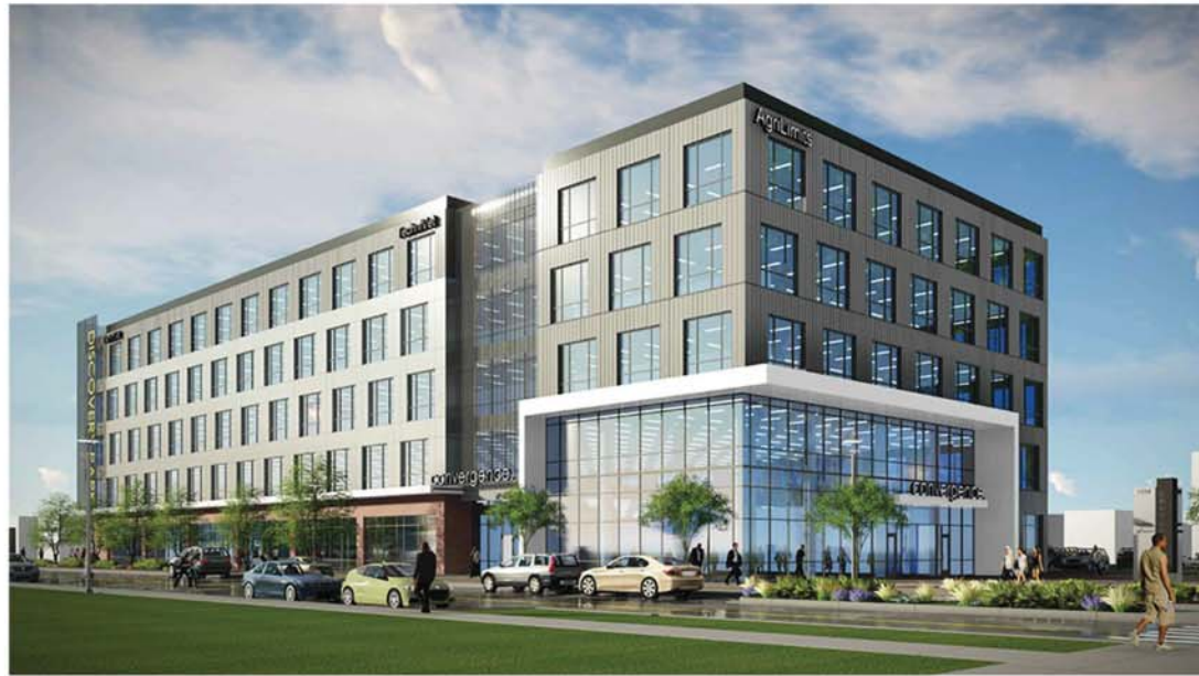
South West View
